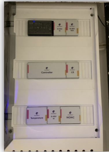
5. 5 - Ready mountable low-current Chameleon distributor
